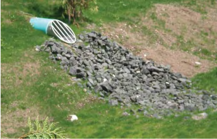
This energy dissipator is in good condition.
