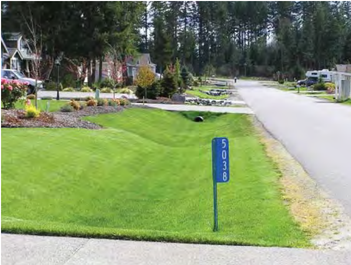
A well-maintained swale
