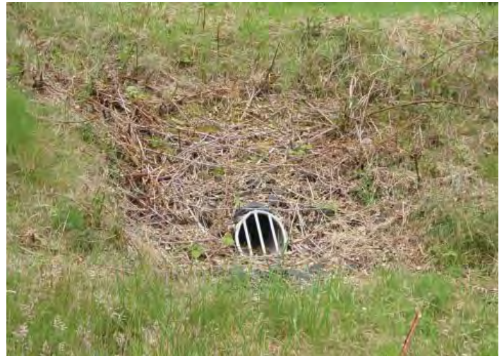
A typical outlet pipe
