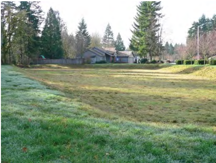
A well-maintained dry pond.
