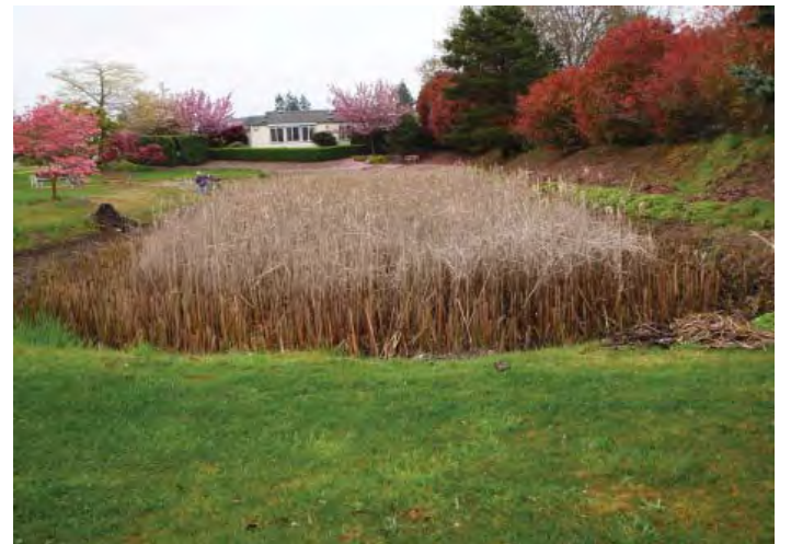
This wet pond is overgrown with cattails.
